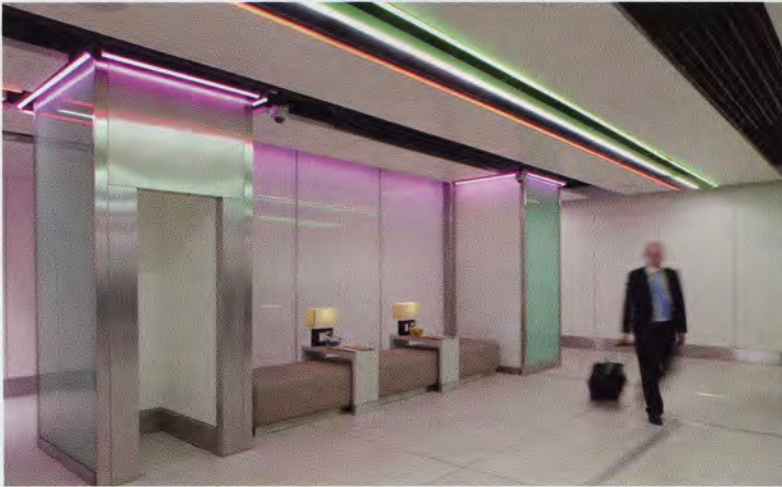
Search and rescue The new linear lighting system, which incorporates LEDs, T5 luminaires and colour-coded columns, helps passengers to quickly navigate their way through airport security.
