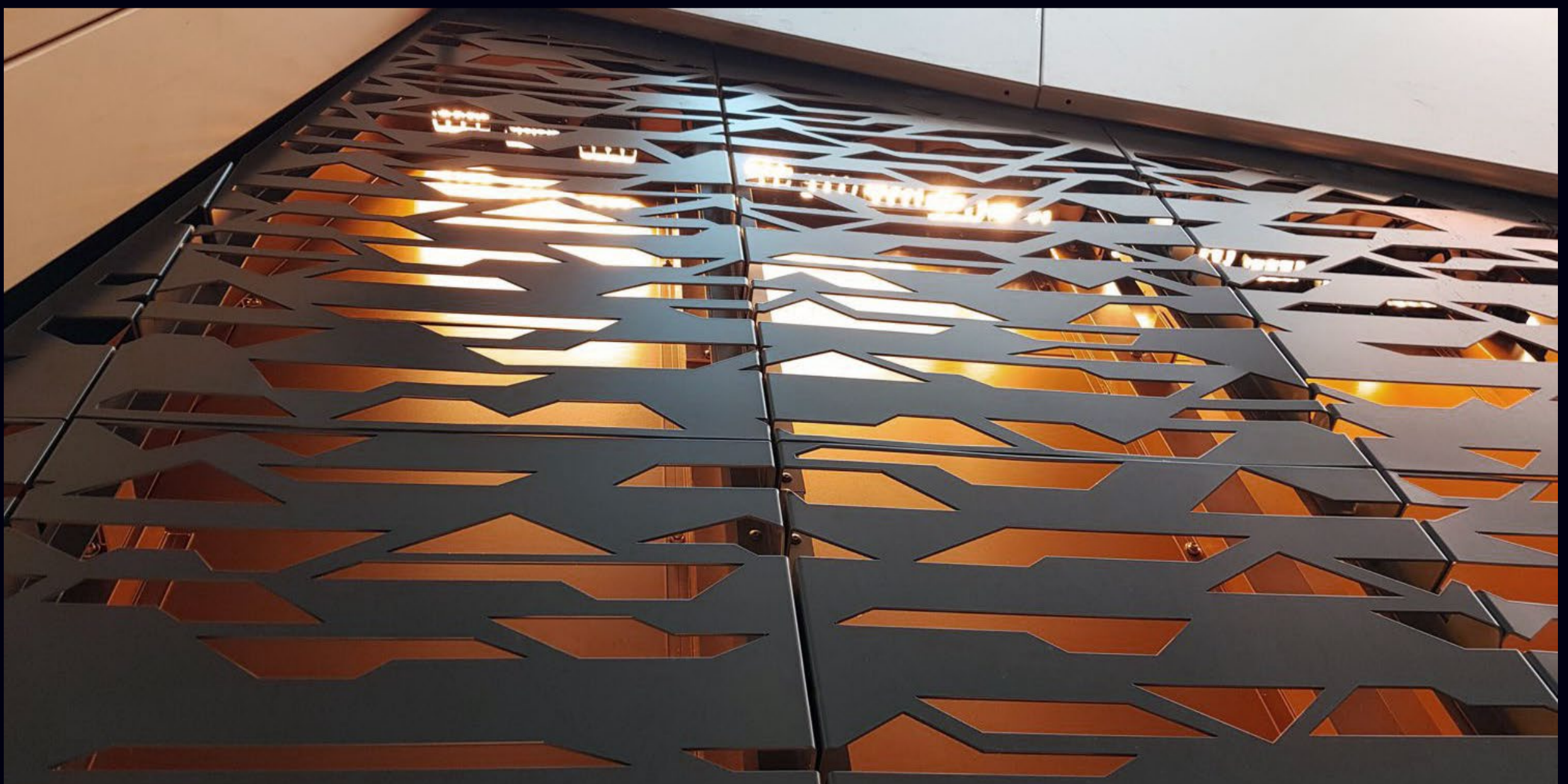
Lakeside Shopping Centre, UK Lighting design by Hoare Lea
